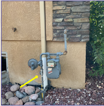
The main gas shutoff valve.
