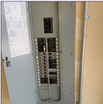
The main electrical service panel.
