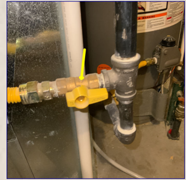
The gas shutoff valve.
