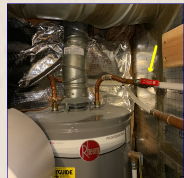
The Water Heater water shut off valve.
