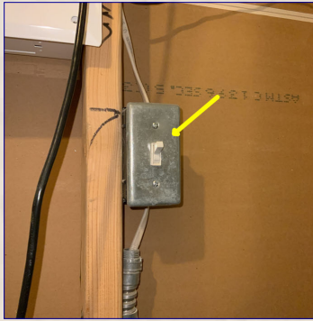
The electrical shutoff switch.
