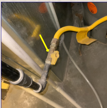
The Water Heater gas shut off valve.
