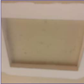
The Attic Access View
