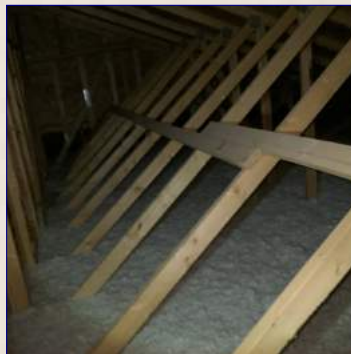
The Attic View
