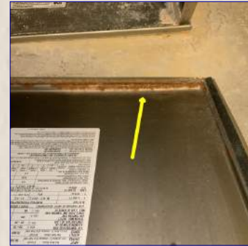
The furnace showed signs of rust and corrosion. Recommend a professional HVAC technician evaluate and repair as needed.
