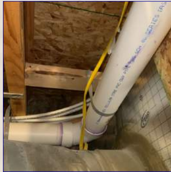
The visible drain/waste piping.
