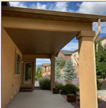
The Deck/Porch/Patio Cover View
