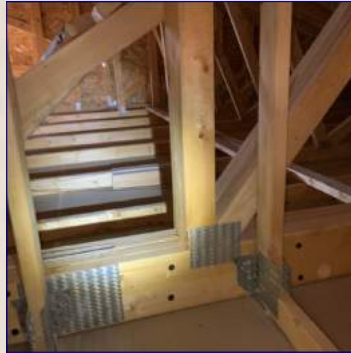
The Attic View
