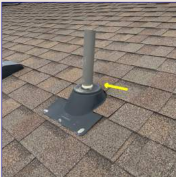
The Plumbing Vent(s)
