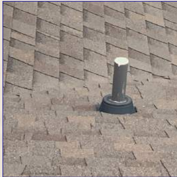
The Plumbing Vent(s)
