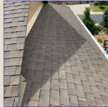
The Roof View
