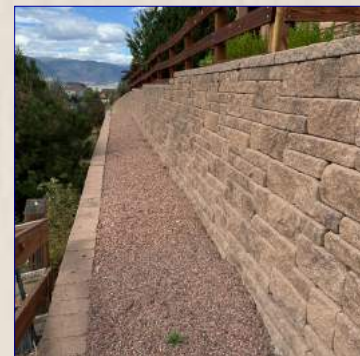
The Retaining Wall View
