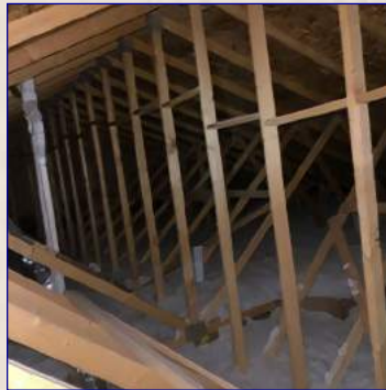
The Attic View
