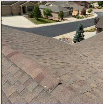
The Roof View
