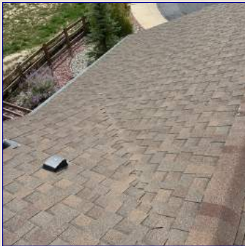
The Roof View
