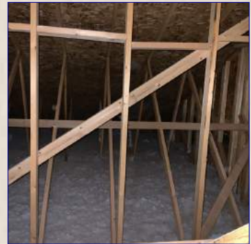
The Attic View
