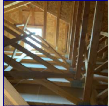
The Attic View
