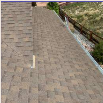
The Roof View
