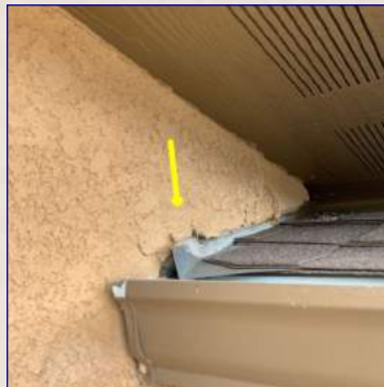
Kick Out flashing is missing at one or more locations, which may allow moisture damage on the home's exterior, walkways, and driveways. Recommend a licensed contractor install flashing to help properly move water to the gutter system. Repair damaged areas as needed.
