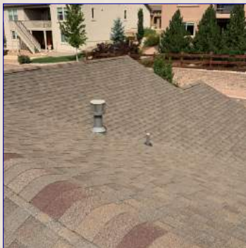
The Roof View
