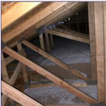
The Attic View
