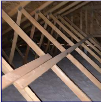
The Attic View
