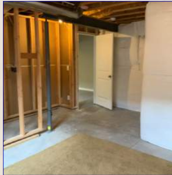
The Basement View
