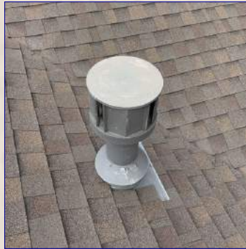
The Chimney Chase
