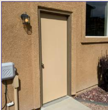
Garage exterior service door view.
