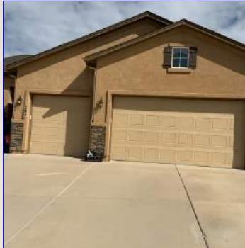
Garage overhead door view.
