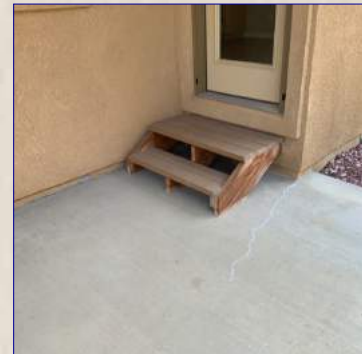
The Steps/Stoop View
