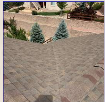
The Roof View
