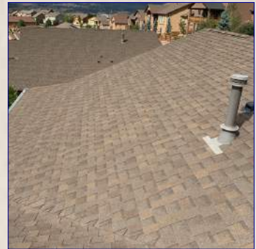
The Roof View
