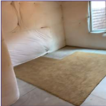
The Basement View
