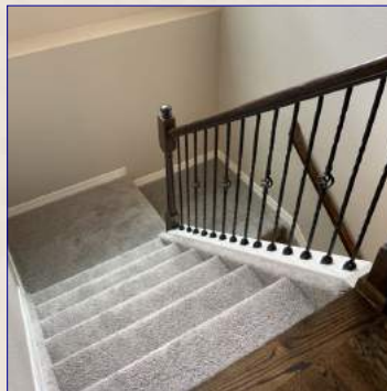
The Interior Stairway View
