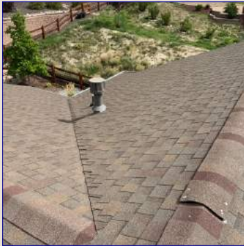
The Roof View
