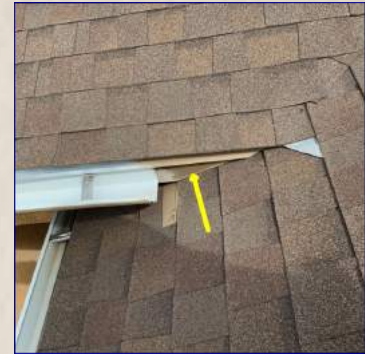
The fascia needs routine painting maintenance. Recommend a professional painter repair/paint the fascia.
