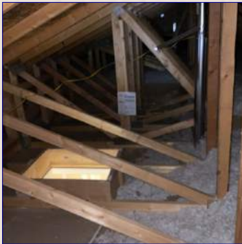
The Attic View
